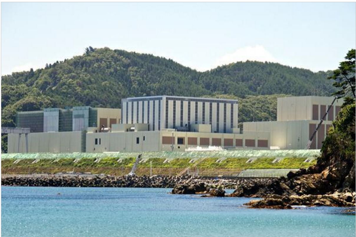
The Onagawa nuclear power plant in Miyagi Prefecture. Tohoku Electric Power will shut down the No. 2 reactor around Saturday because a valve in equipment connected with the feedwater system is leaking about 0.2 tons of water an hour; the company says the surrounding environment is unaffected. (File photo: WPM Productions)
