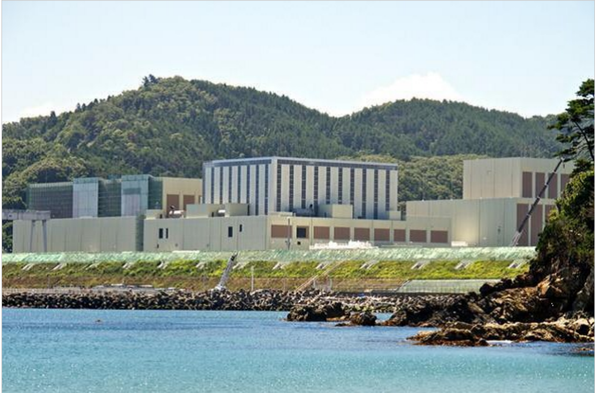
The Onagawa nuclear power plant in Miyagi Prefecture, in a file photo. Tohoku Electric restarted the No. 2 reactor on Monday after replacing a valve that had leaked water containing traces of radioactivity. (File photo: WPM Productions)
